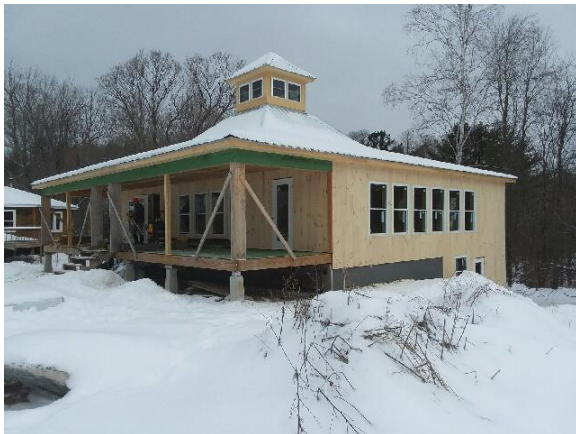
The siding has just been finished— photo by Kingdom Construction
