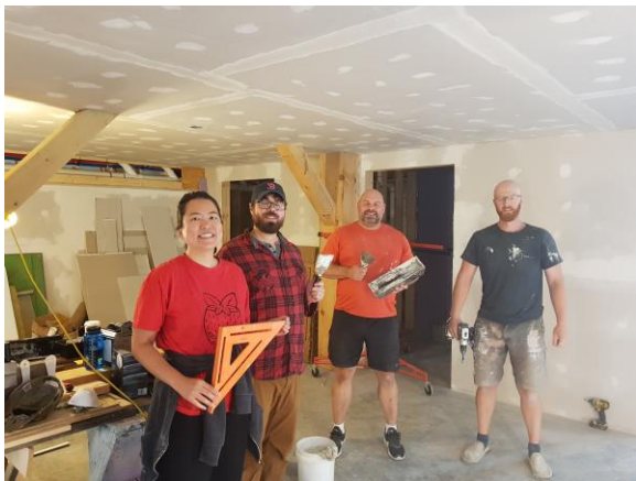
And the ceiling is finally sheet rocked
