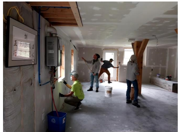
Painting the basement in the dining hall
